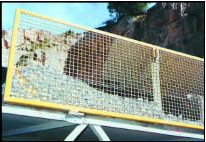
Example of a hinged guard which swings downwards
